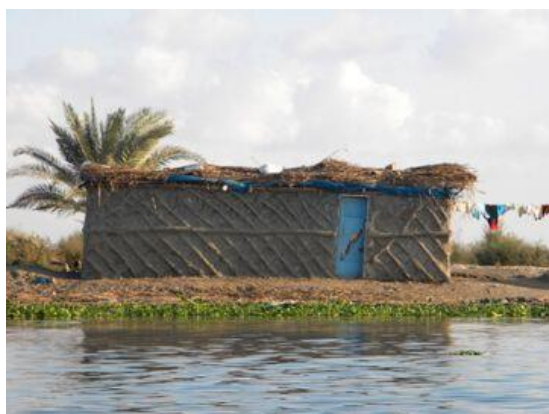
Fig (8) A crudely applied mud mortar (the mud of the lake is black, and making the hut appear dull grey when dry) –the dweller admitted that the quality of the hut and the plastering are not as good as they used to be since most of the few remaining huts are used as rest houses or shelters for fishermen.
