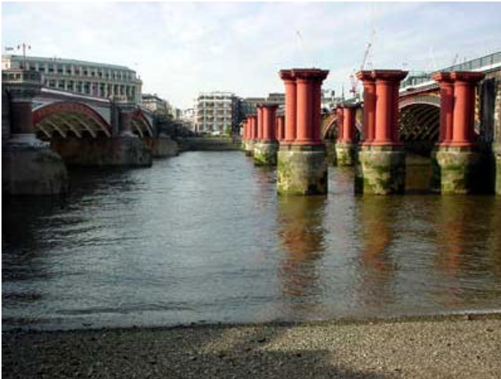
Figure 212. Blackfriars Bridges - Old and New, Vehicular on the Left and Rail Bridge on the Right. Thames - Low Tide.
