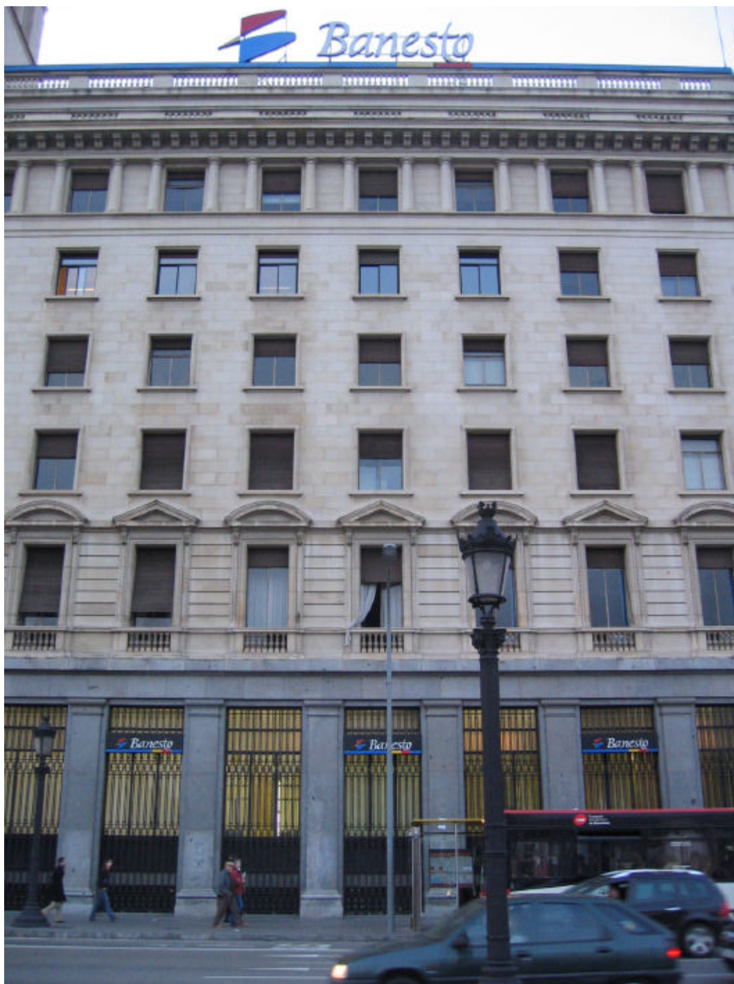
Figure 331. The Banesto Building with No Transparency and No Accessibility. The only activity is usually people waiting for the bus
