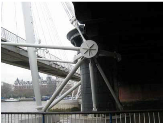
Figure 194. The Structure of the New Pedestrian Bridge Attached to the Old.
