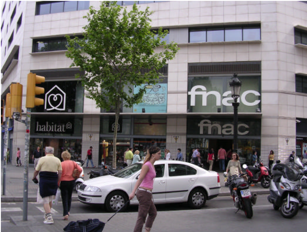
Figure 332: El Triangle Commercial Centre in the intersection with Carrer Bergara, featuring high levels of transparency and a big accessible space
