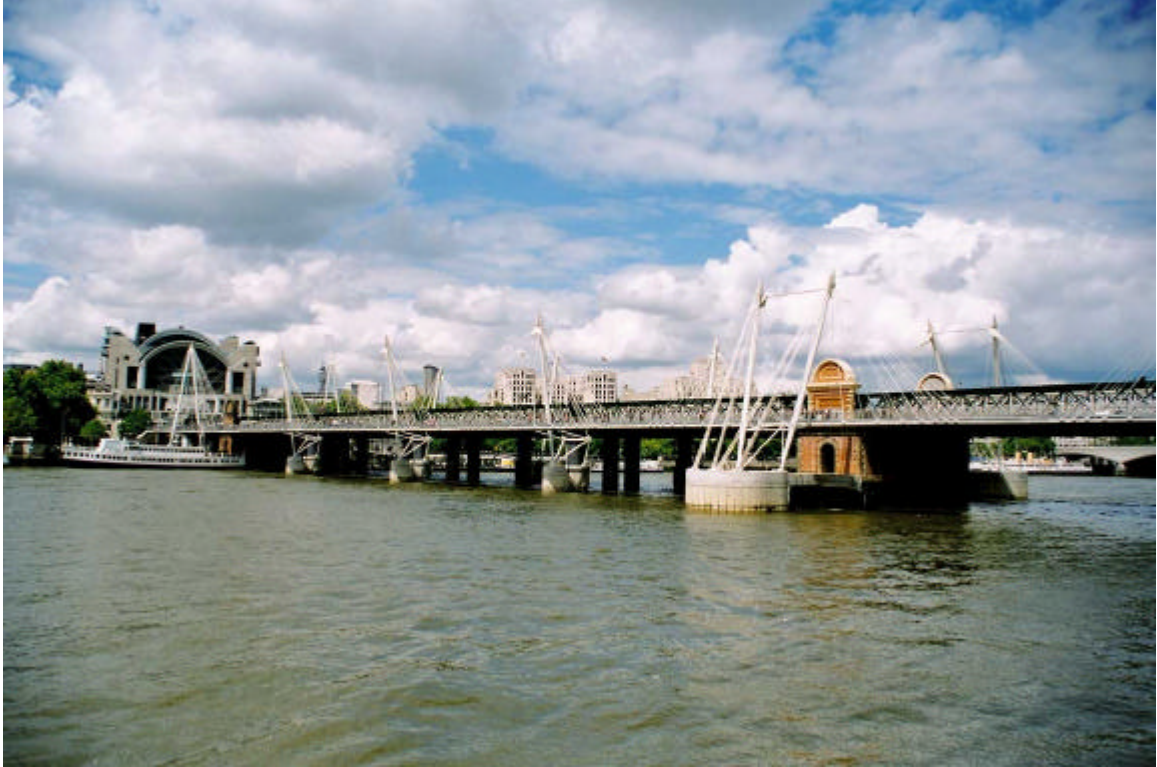
Figure 193. The New Pedestrian Bridge Viewed From the Southbank.
