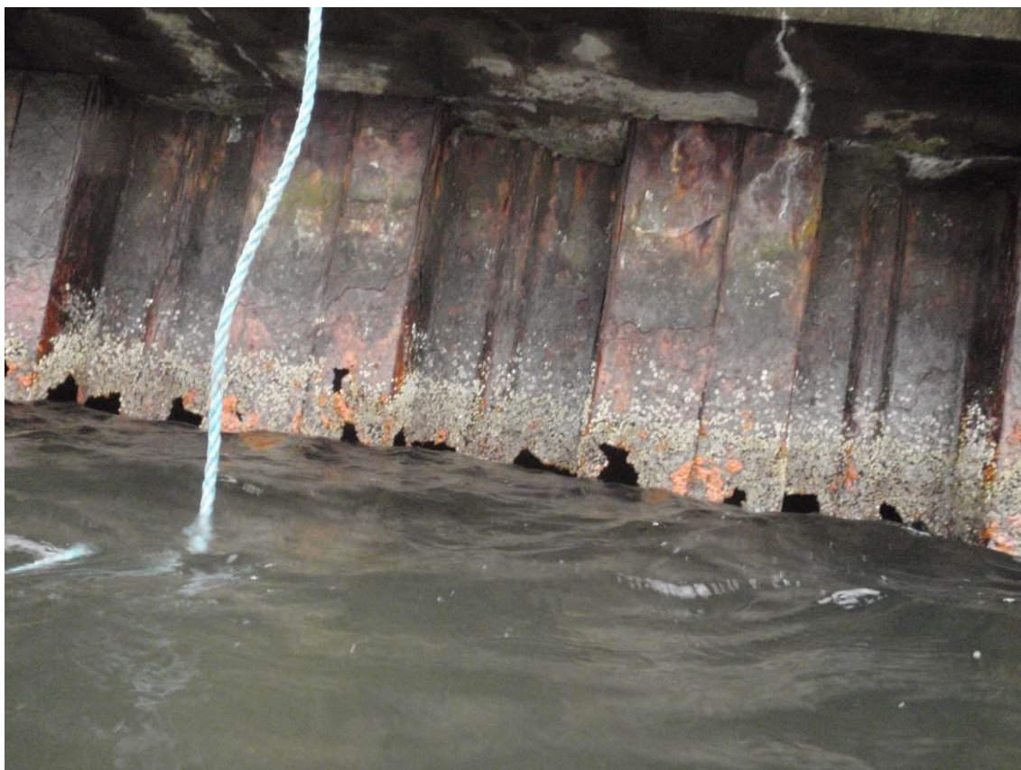
Figure 1: Sheet pile wall on the Swedish east coast suffering from severe corrosion (Joakim Brogstam, MarCon Teknik AB)
