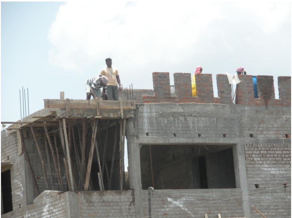
Figure 12: Picture from the construction site.
