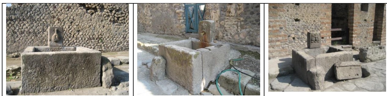
Figure 3.2 a, b and c. Street fountains nos. 20, 21 and 27 with basins. Photos by author. The overflow outlet is clearly seen in 3.2 b, as is the outlet for cleansing at the bottom.
