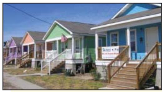
Some of the first houses erected at the Musicians' Village site.
