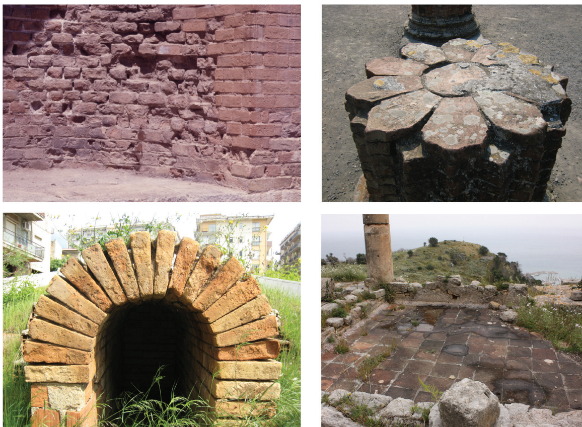
Figure 4.1. Hellenistic fired bricks (Tauromenion, Pompeii, Rhegion, Soloeis). Photos by H. Gerding.
