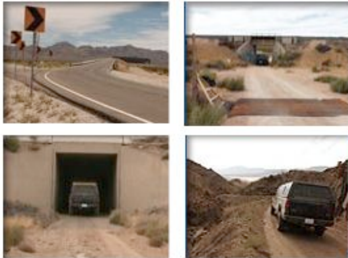
Figure 49: Four challenges on the GCE course; (from left to right, top to bottom) railroad overpass, cattle guard, 150-foot long tunnel, mountainous road. The locations off the challenges are shown in the map above (marked as B, G, H and K).
