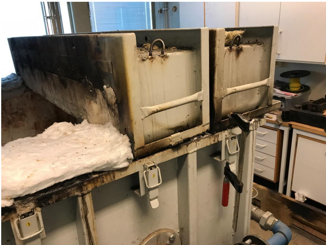
fig. G-18. Steel beams with ceramic insulation placed on the top of the furnace.
