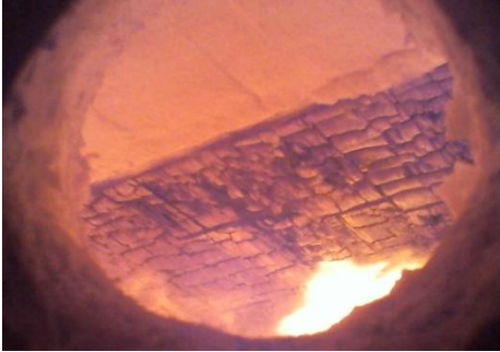
Initial stage of delamination
