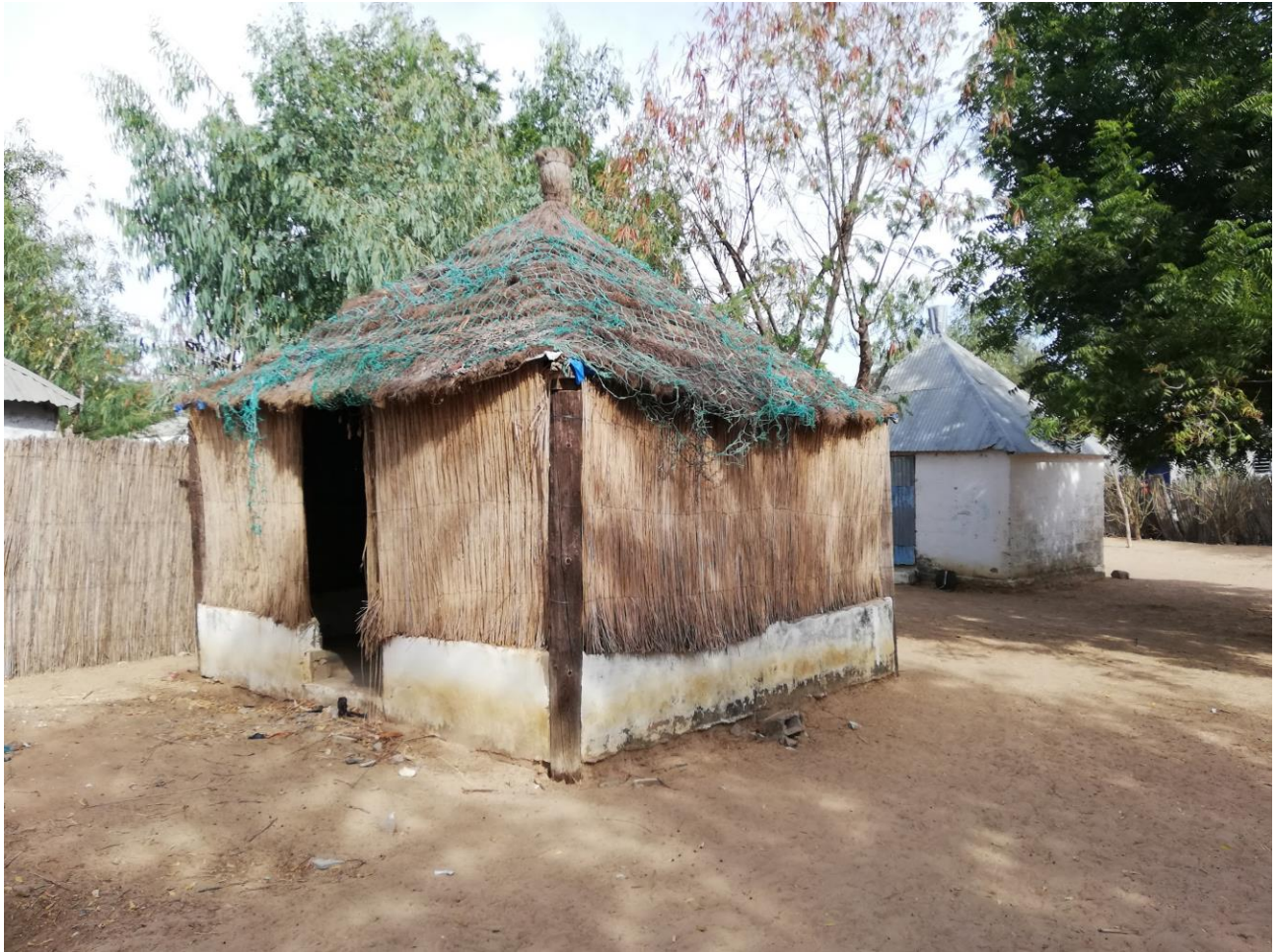
Figure 3: Straw and concrete huts in Ndem
