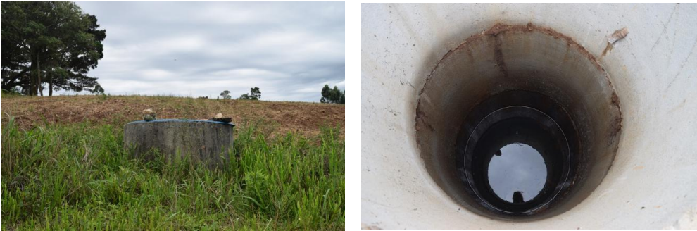
Figure 44 and Figure 45. Groundwater well and storage tank of São Domingos
