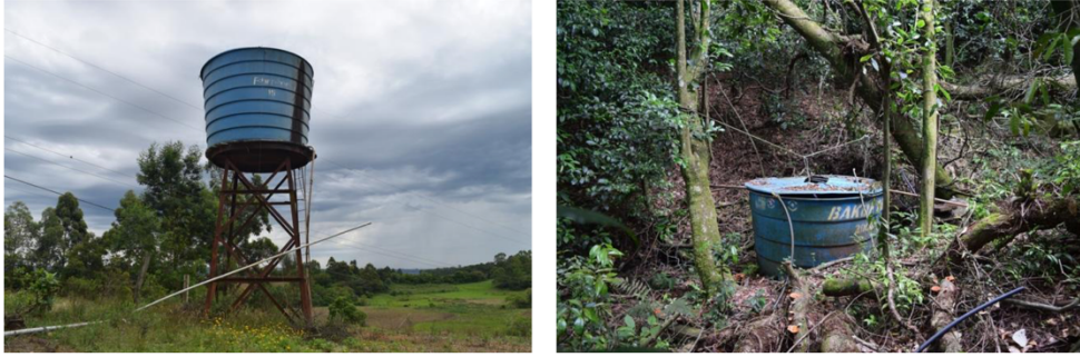
Figure 46 and Figure 47. Water tower and water storage tank of São Domingos
