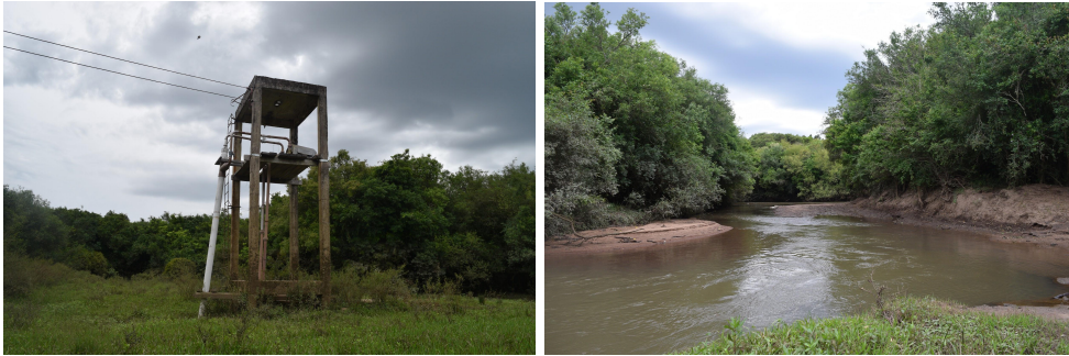
Figure 38 and Figure 39. Arroio Turuçu and the pumping construction of the SAA system.
