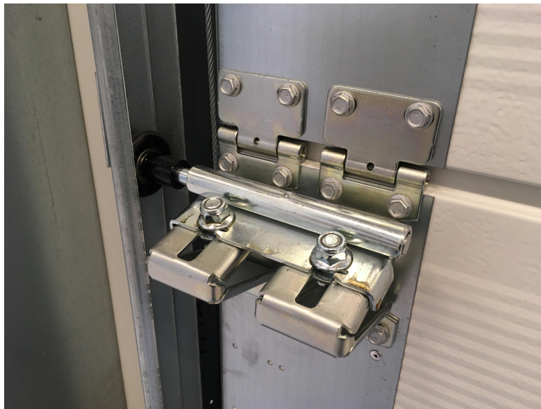
Figure 2.1: J-Track holding one of the door rollers in place. The door roller is fixed on a hinge which connects two door sections.
