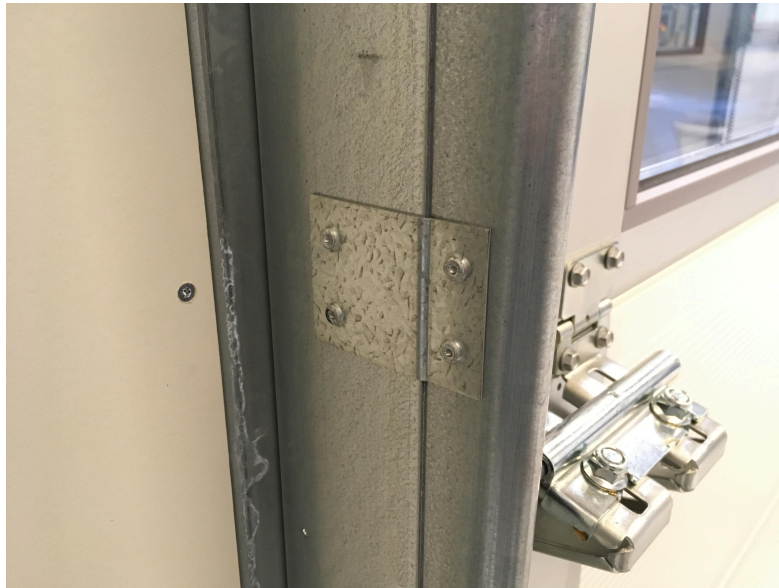
Figure 6.8: A current connector plate. Note how the geometry of the connector plate connects the wall bracket and the vertical J-Track.
