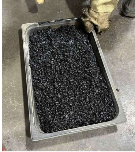
Figure 3. Freshly mixed asphalt.
