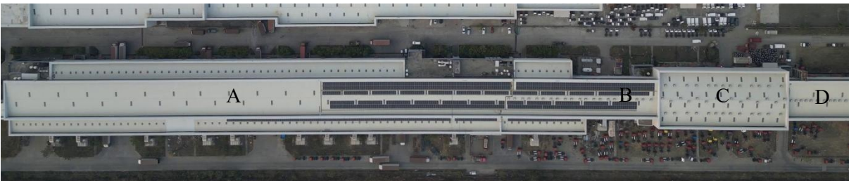
Figure 42. Aerial View (Top): Assembly Shop
