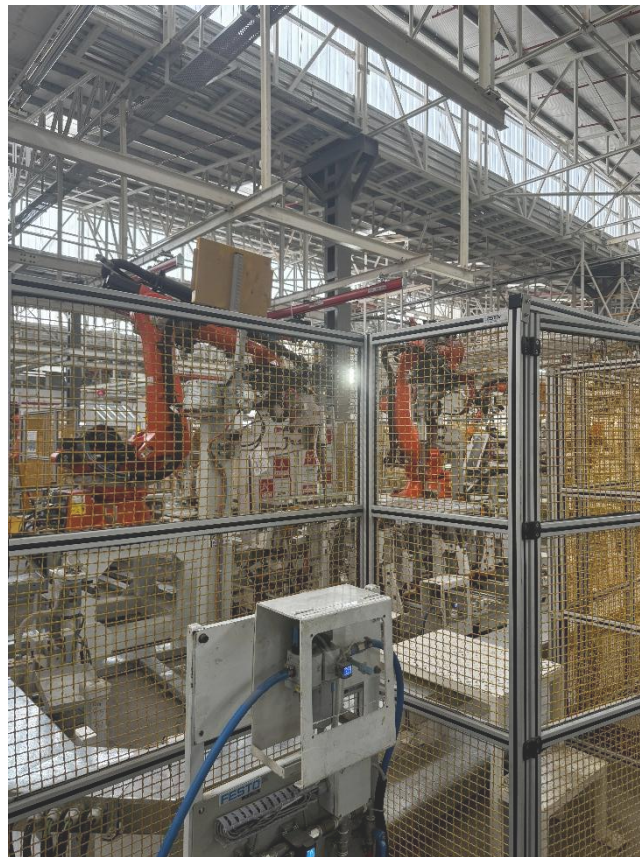
Figure 47. Weld Shop: Interior showing northbay and roof skylights.
