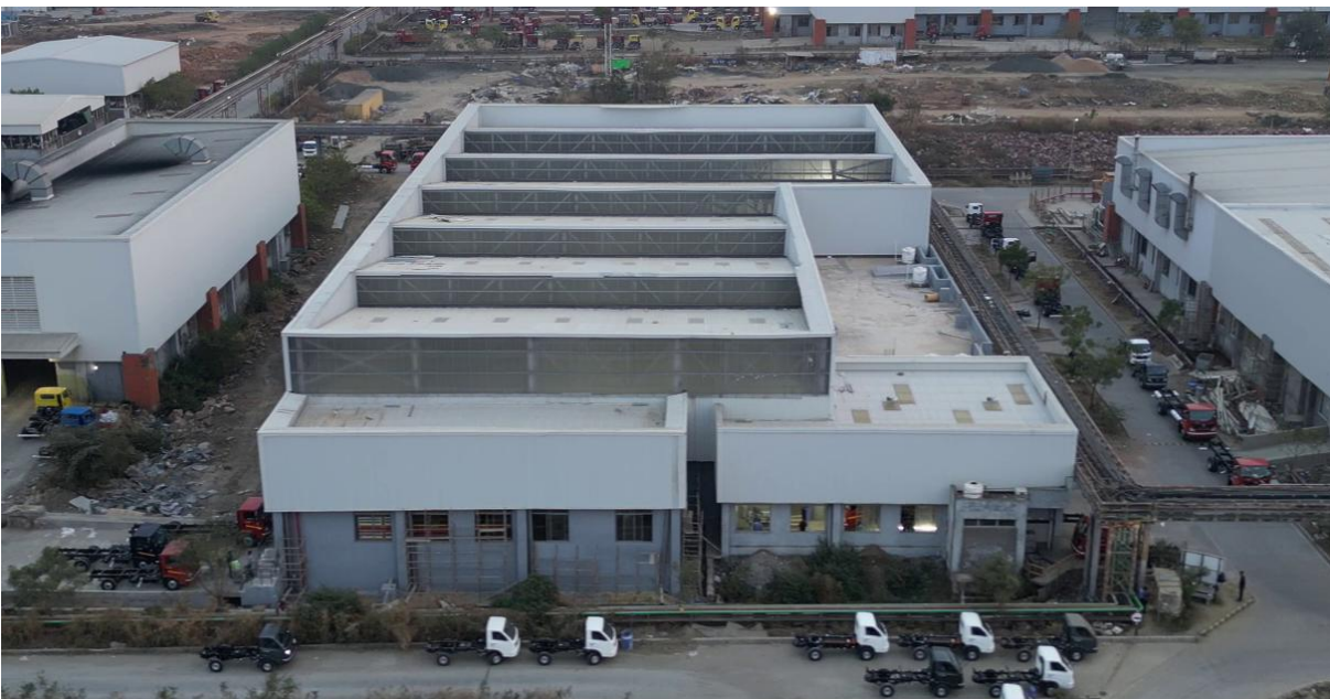
Figure 43. Aerial View (North): Machine Shop
