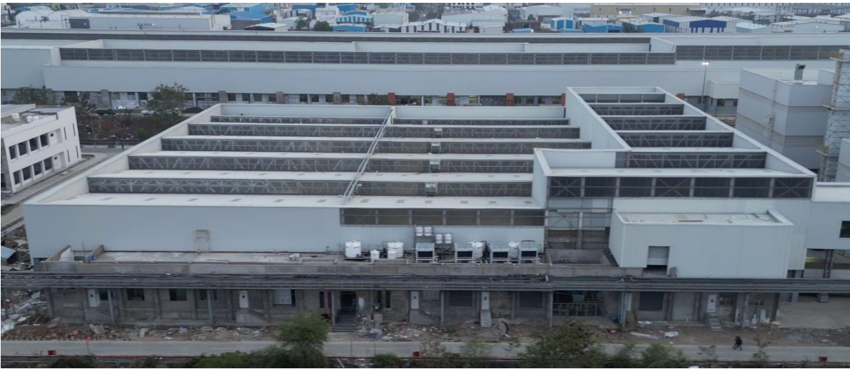
Figure 44. Aerial View (North): Weld Shop
