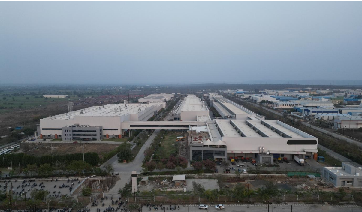
Figure 41. Aerial View (West): Industry campus
