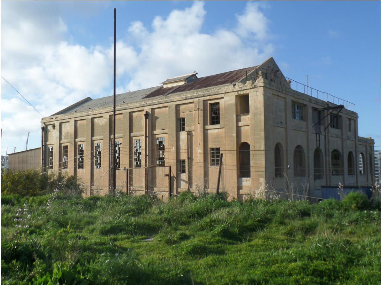
Figure 7. An abandoned building on Manoel Island from my field journal. Source: Own Photograph, 2026.
