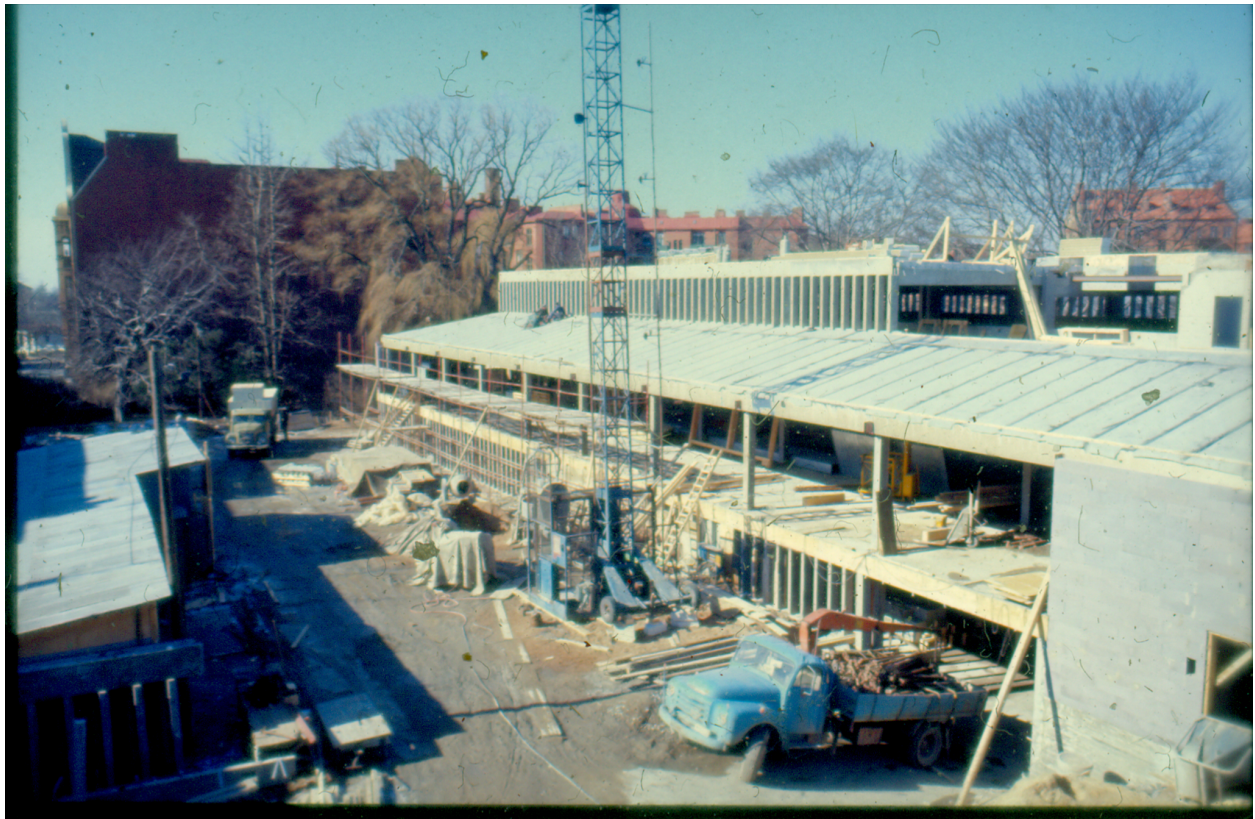
Figure 1. Construction of the City Library, 1969. (Source: Lunds Stadsarkiv)
