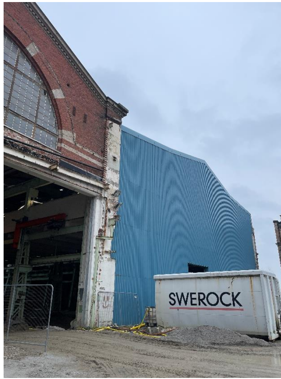
Figure 9 The state of the south façade during the site visit
