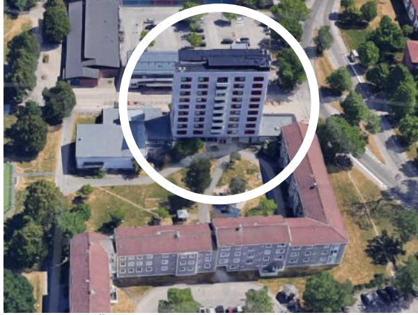
Figure 8 Örebro - high-rise multi-apartment building.
