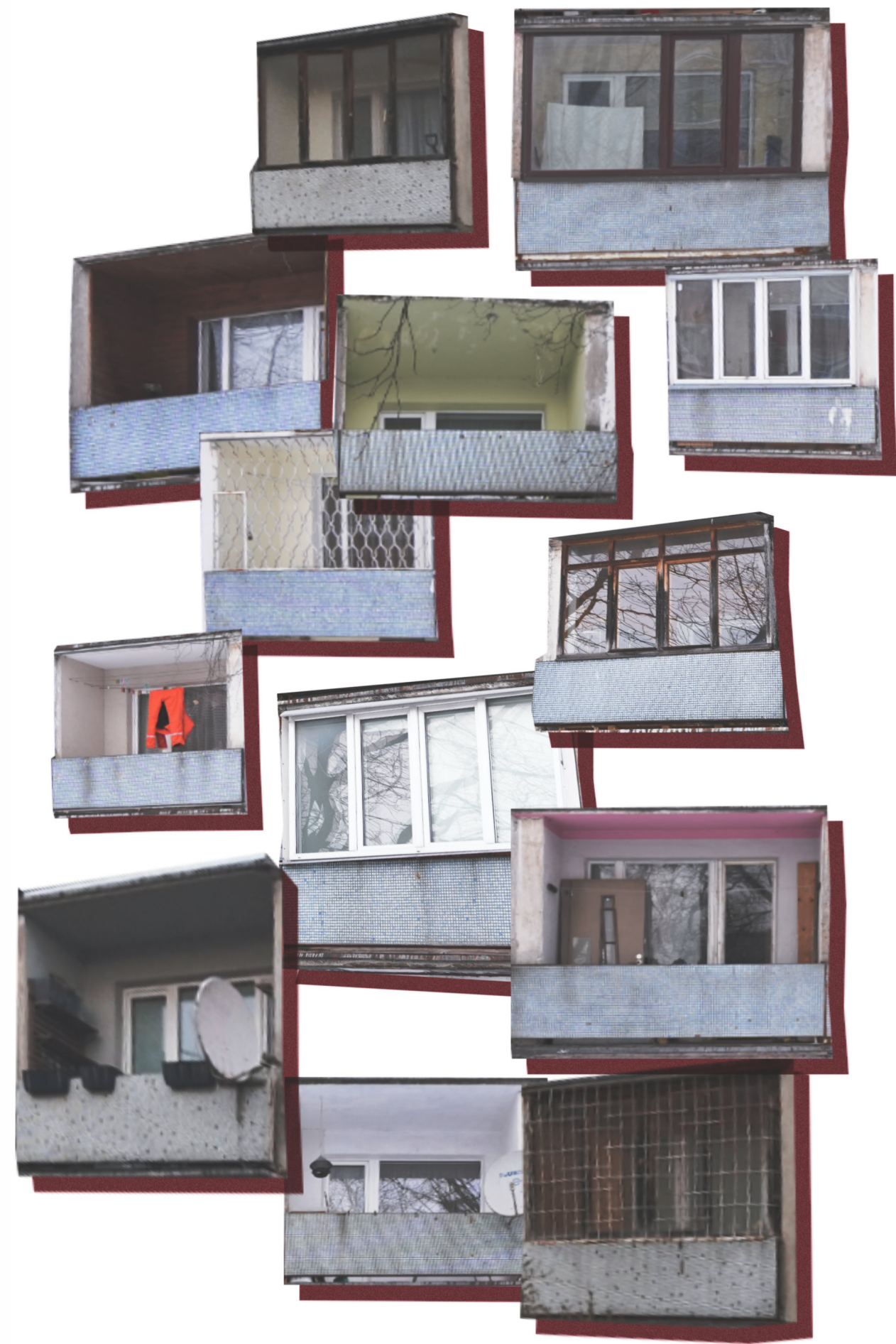
Figure 5. Different ad-hoc loggia solutions in 1-464A series buildings in Ilūciems
