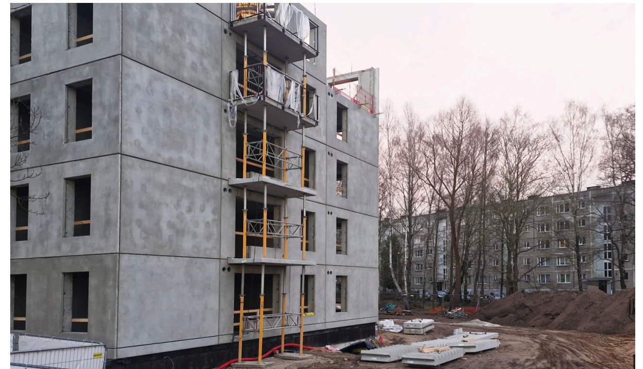
Figure 22. A new construction currently ongoing in Iļģuciems, with series 1-464A residential buildings in the background
