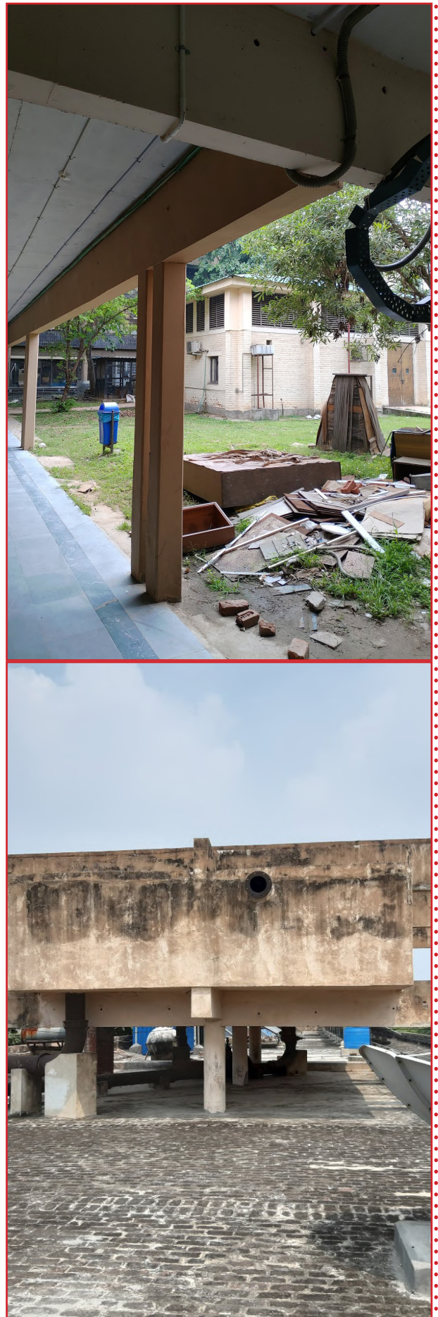
Fig 23 Images of Academic Block 3 at IIT Delhi, one of the oldest buildings in the campus.
