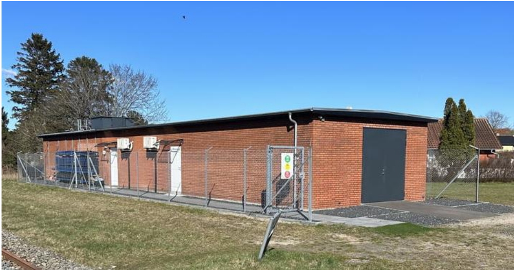
Figure 4.2. Kirke Eskilstrup Waterworks Pump Station/Office
