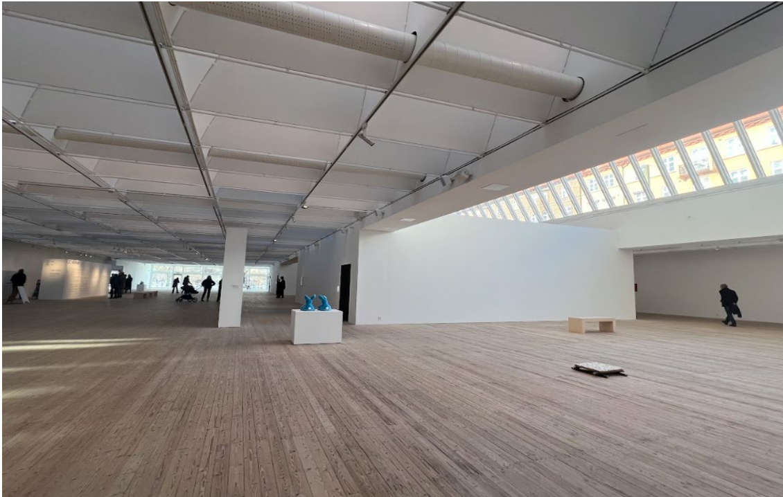
Figure 8. Interior view illustrating the open exhibition space and the influence of layout and internal elements on daylight distribution (author's own photograph)
