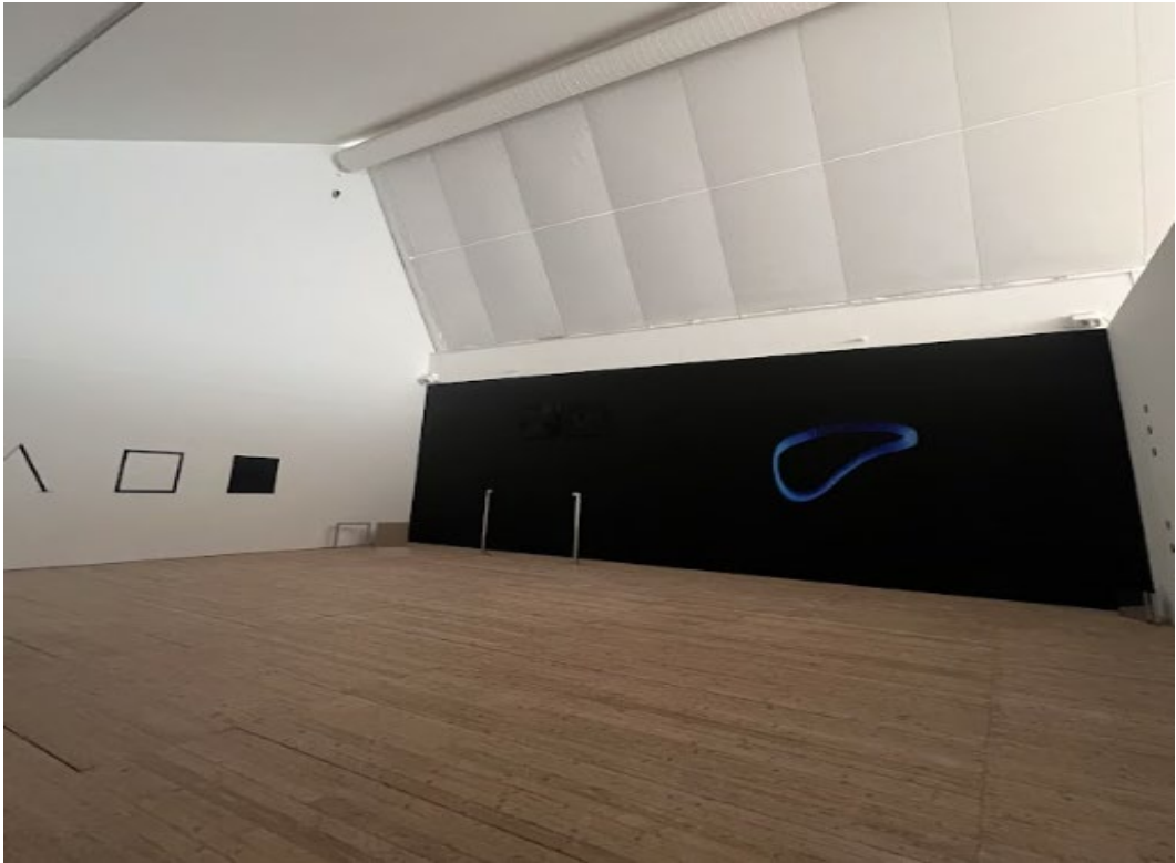
Figure 48. Interior exhibition space showing partially covered skylight openings used to control daylight penetration
