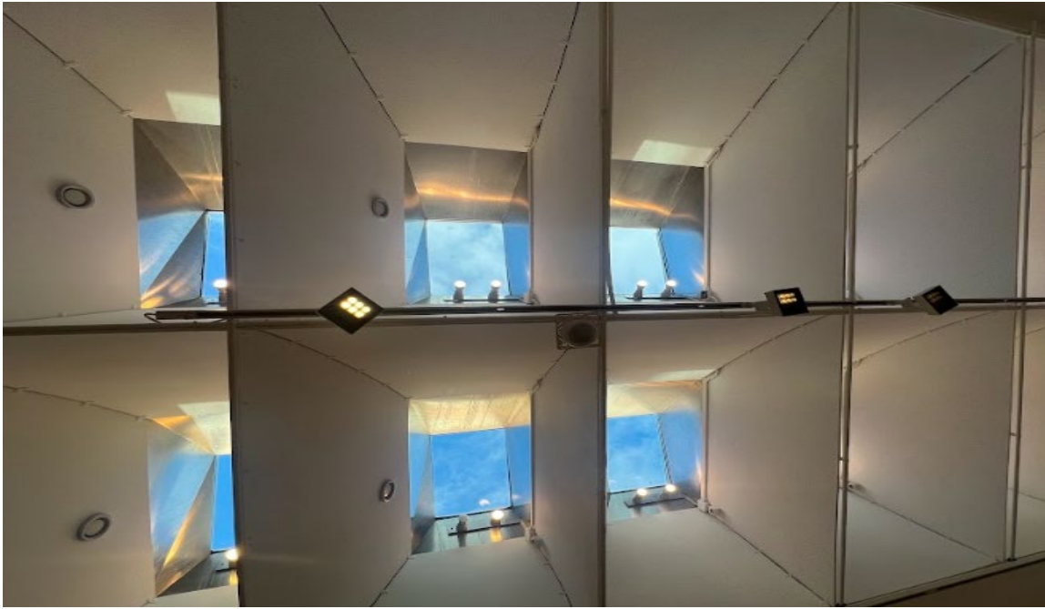
Figure 6. Interior view of the saw-tooth skylights showing diffuse daylight and internal reflections within the roof structure (author's own photograph)
