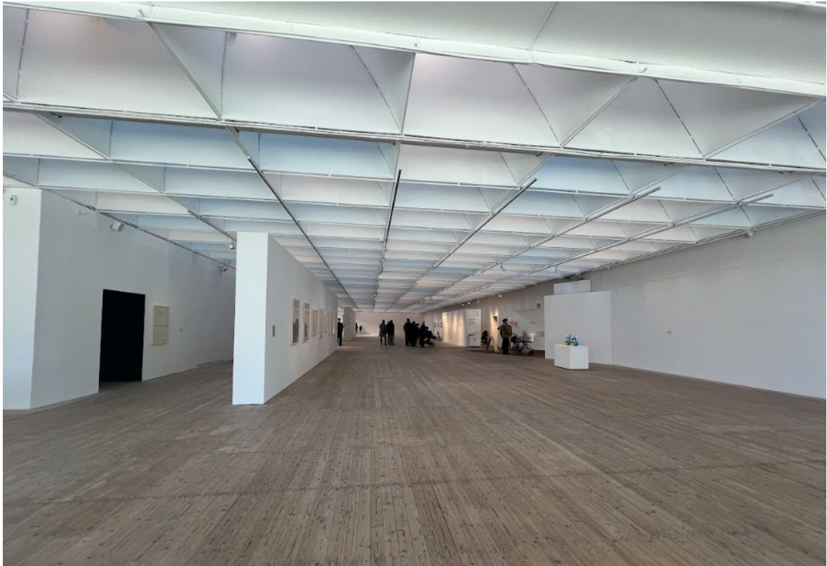
Figure 51. Main exhibition hall with diffuse daylight distribution from the ceiling system
