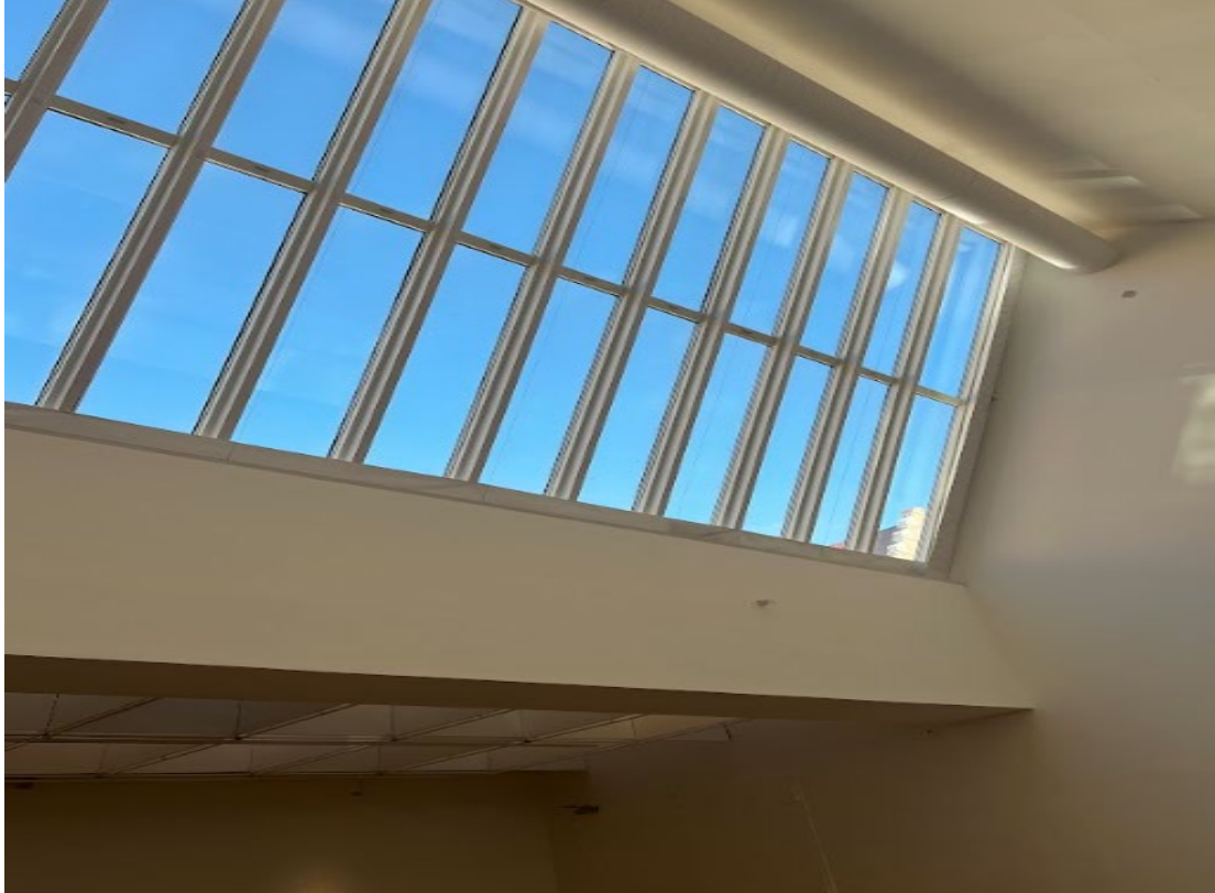
Figure 49. Large skylight glazing system providing daylight penetration into the exhibition space
