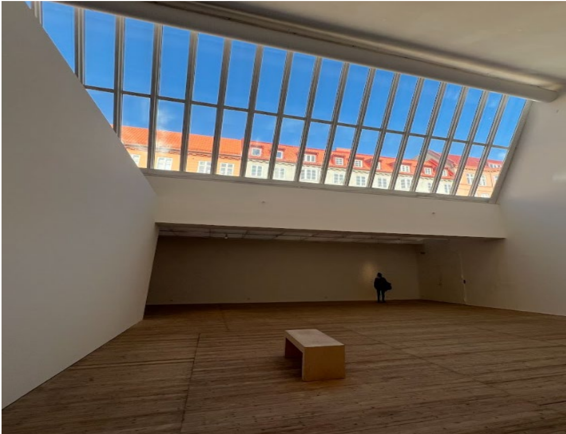
Figure 50. Exhibition hall showing daylight distribution from the large skylight glazing
