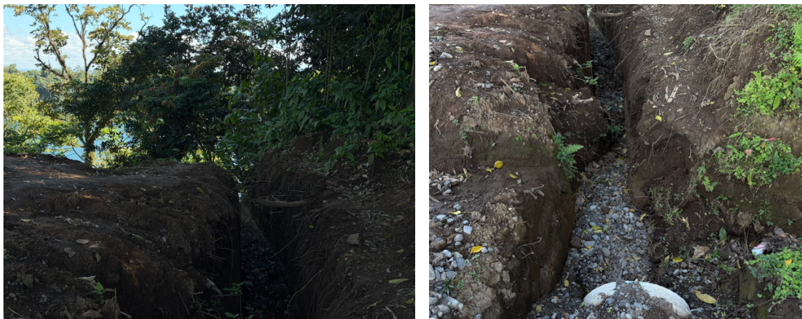
Figure 2.5 and 2.6: Observed drainage channels located on the western slope of Río Cuarto Lake, directing surface runoff toward the shoreline of the lake. A small, constructed tunnel structure can be seen on the left picture at the bottom.
