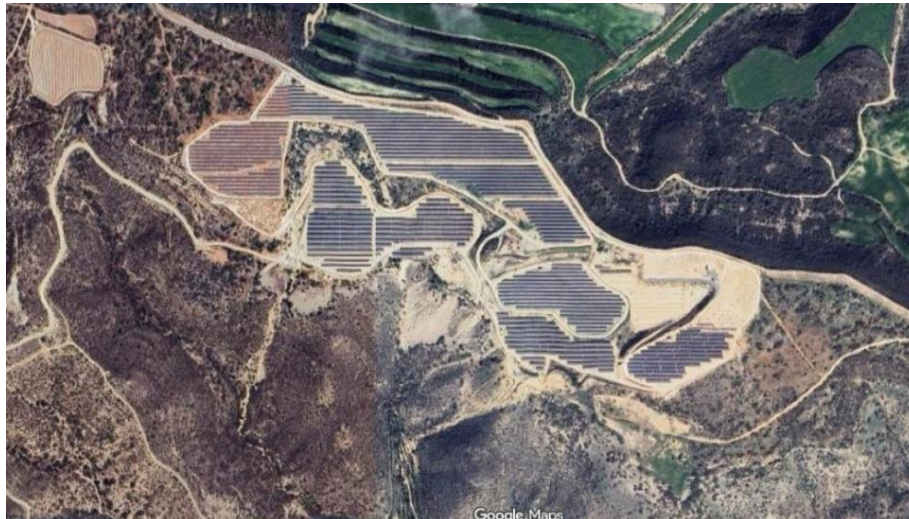
Fig. 1.4: The solar PV installation in Vassiliko, Cyprus. Source: Google Maps
