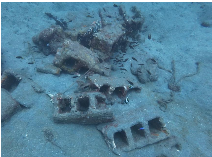
Figure A10: broken concrete artificial reef structure
