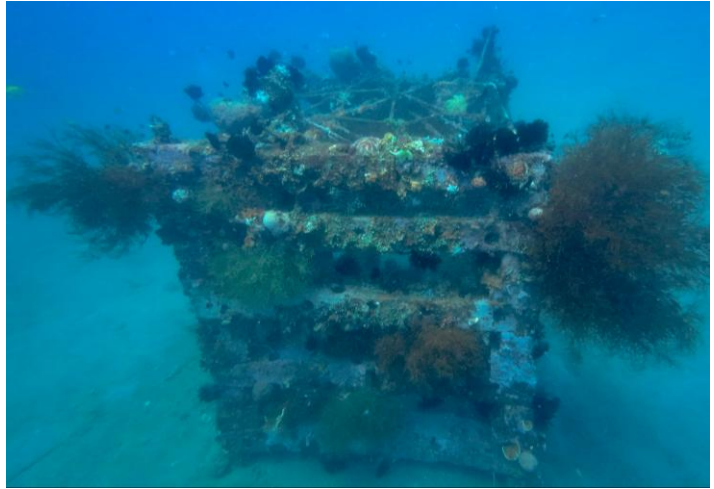
Figure A2: Concrete AR structure 18 years
