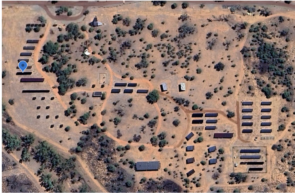
Figure 8: Satellite picture of Australia solar site. The blue arrow indicates the PV system analysed in this report.
