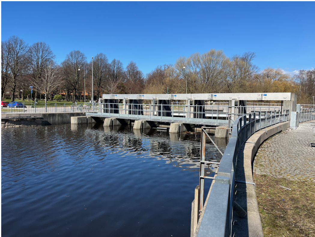
Figure 3.9: Photograph of Gårda dämme from the upstream part. By Vera Åkerlund.
