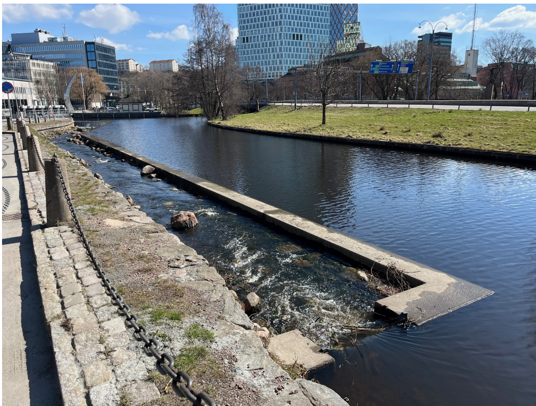
Figure 3.11: Photograph of the fish passage at Gårda dämme. By Vera Åkerlund.
