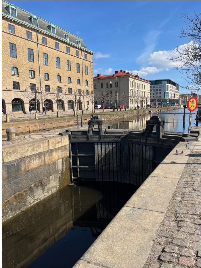
Figure 3.15: Photograph of the canal lock at Slussen. By Vera Åkerlund.
