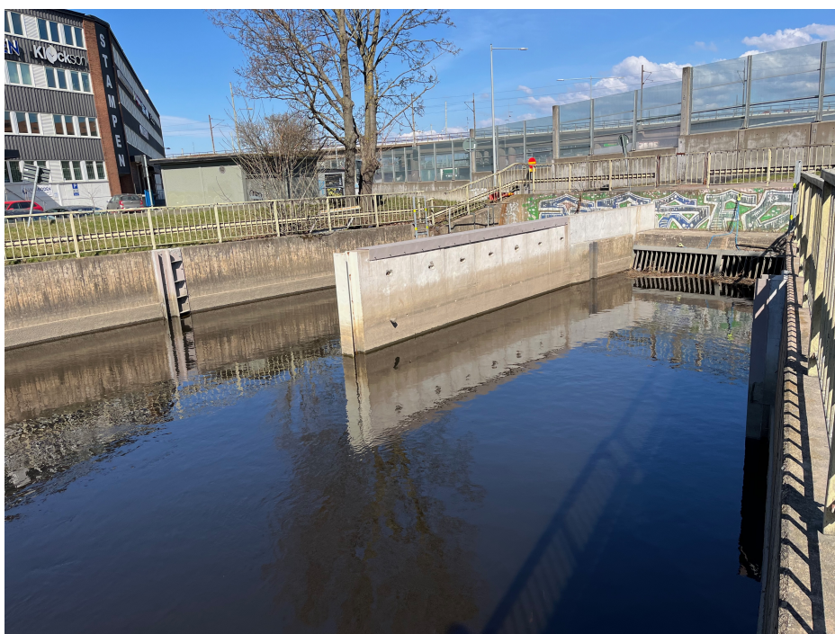
Figure 3.4: Photograph of the inlet to the Gullbergsån culverts. By Vera Åkerlund.
