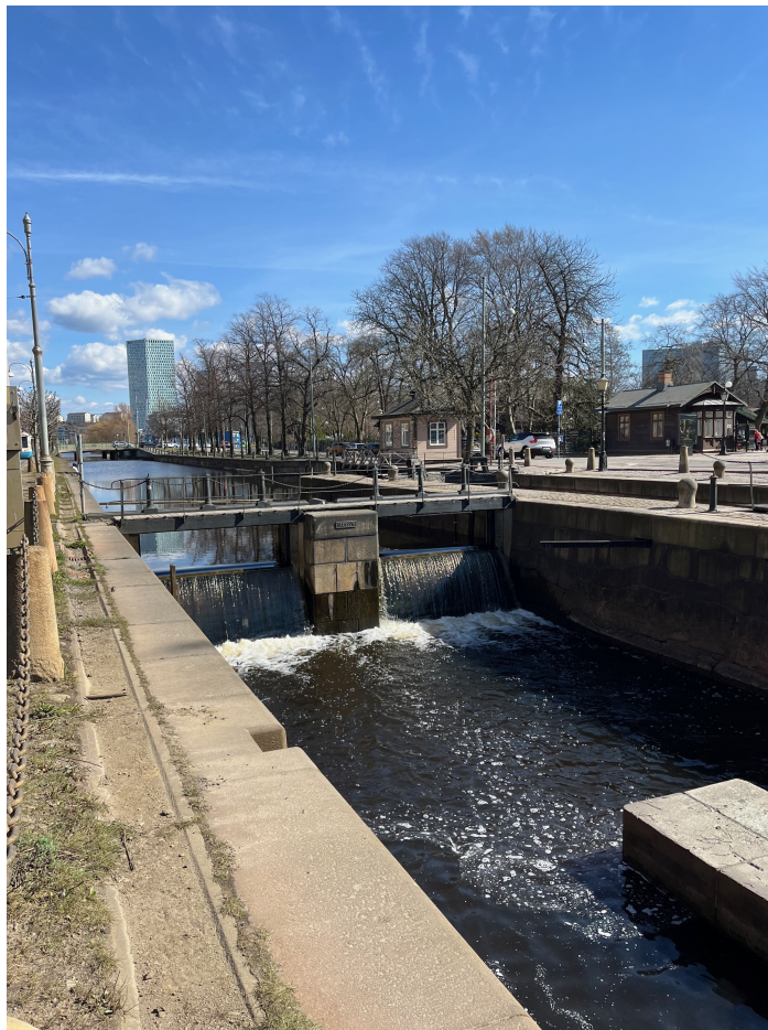
Figure 3.14: Photograph of the regulating structure at Slussen. By Vera Åkerlund.
