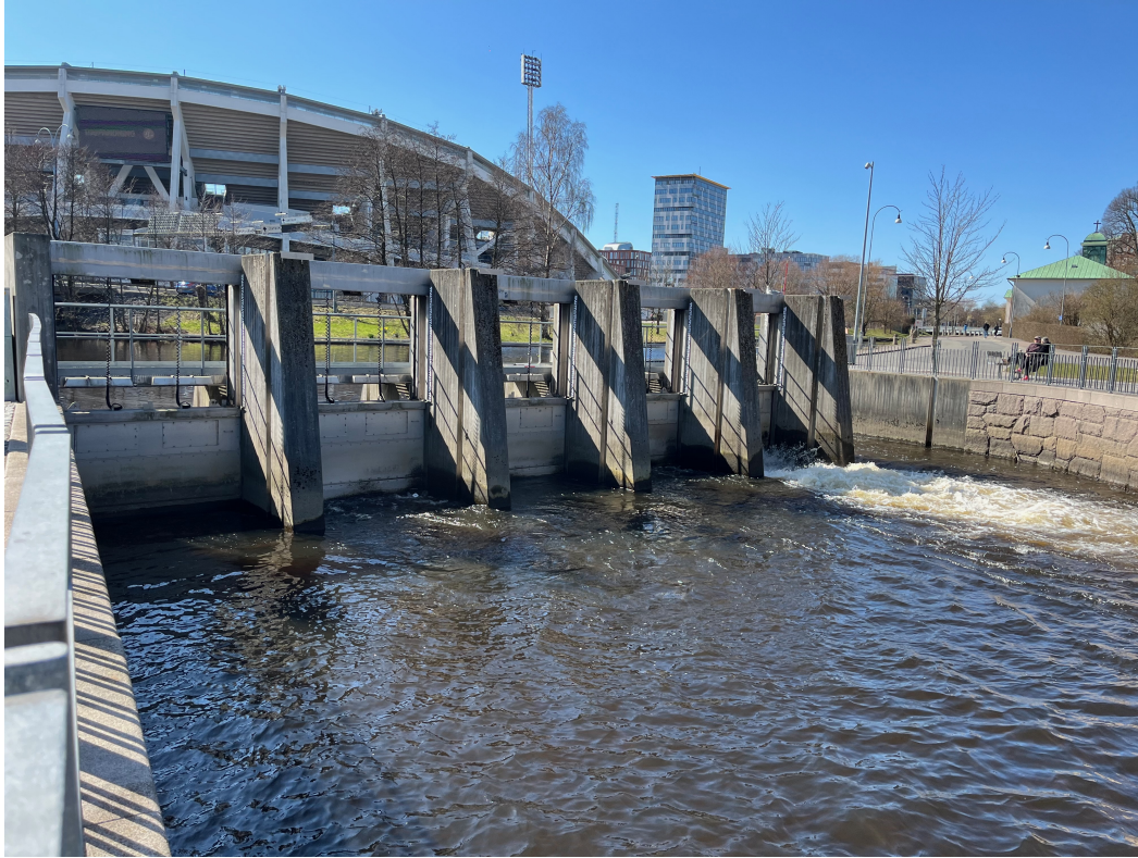
Figure 3.10: Photograph of Gårda dämme from the downstream part. By Vera Åkerlund.
