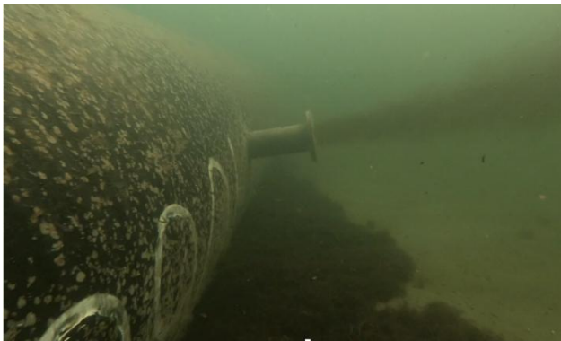
Figures 4-5. Pipes releasing wastewater extending several km underwater, in Nymölla paper mill (left image), and Mörrums pulp mill (right image) (Frilagt, 2019).
