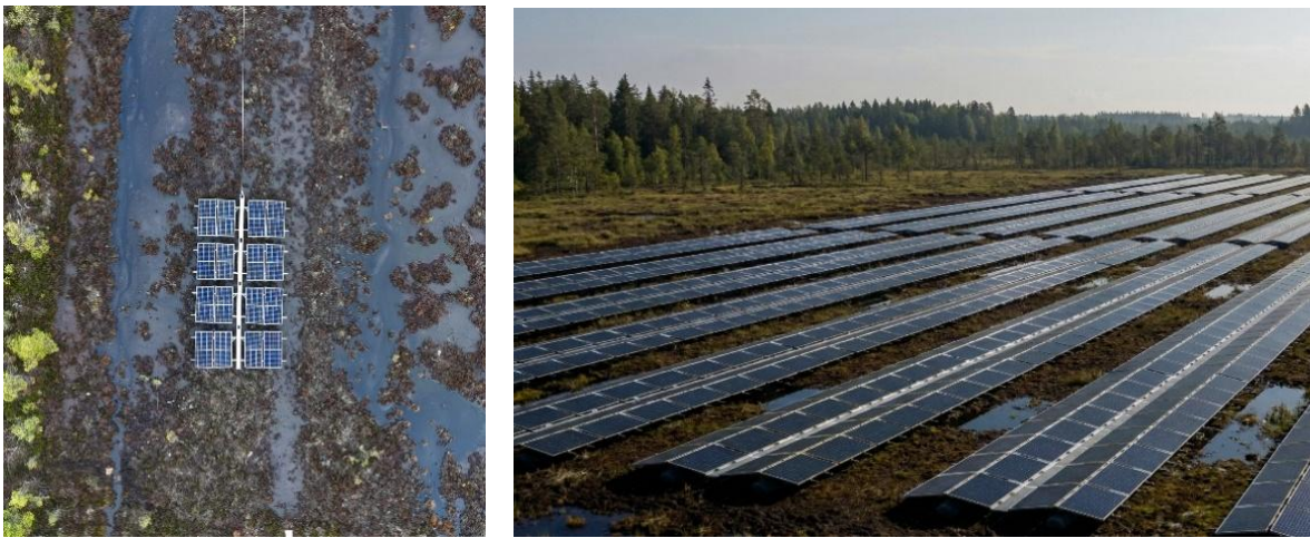
Figure 5-1. Semi-floating solar modules on peatlands
