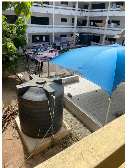
P2 - Water storage tank and informal shade structure
